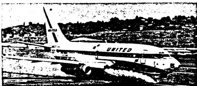
Figure 22. 737-200 Nose Gear Water Spray Testing
